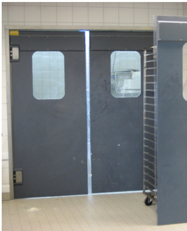
PE bumper above window and PVC finger protection
