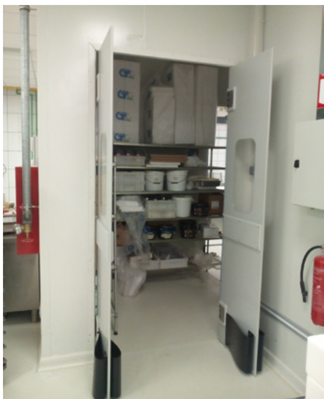
PE bumper and spring bumper
